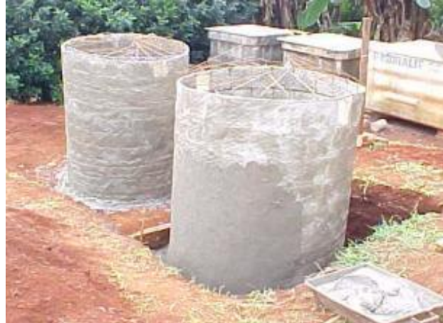
Figure 2: View of RAC under construction Figure 3: Internal view of RAC
