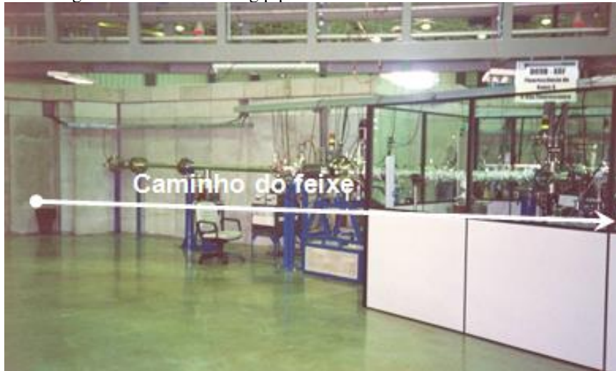
Figure 8: Photo of the ring pipe for the DO9B – XRF line of LNLS.
