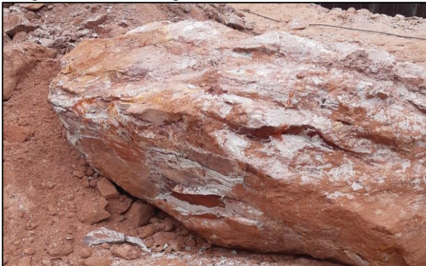
Figure 12. Constant quartzite in the excavation wall
