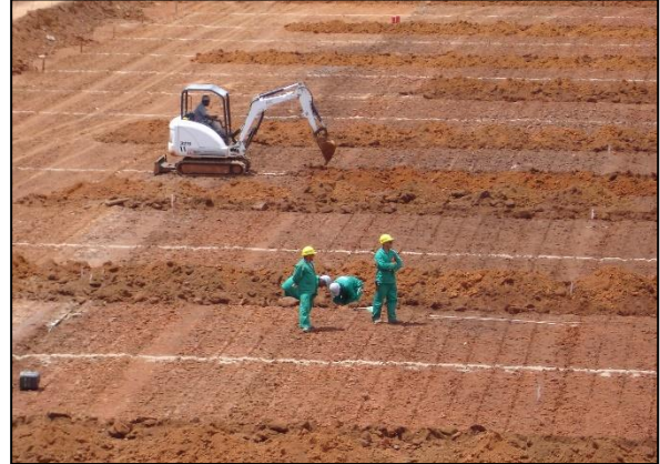
Figure 13. Opening the transverse trenches
