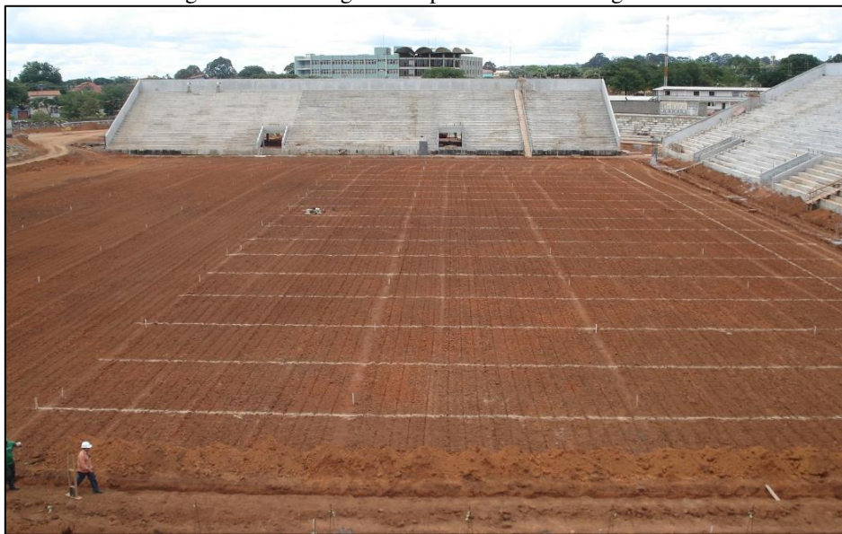
Figure 11. Marking the template for the drainage lines.
