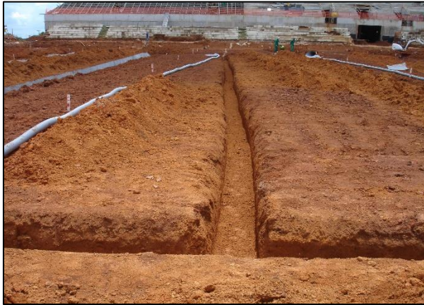
Figure 14. Trenches cleaned for installation of drainage geocomposite
