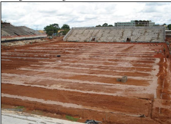
Figure 16. Filling the trenches with washed sand
