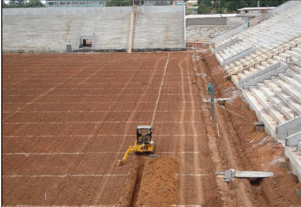
Figure 12. Opening the longitudinal trenches
