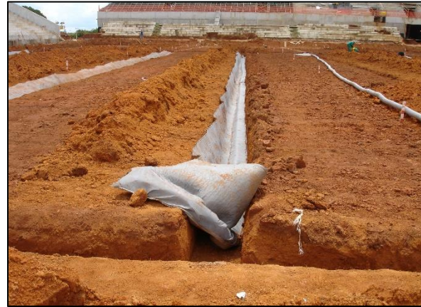
Figure 15. Installation of drainage geocomposite.
