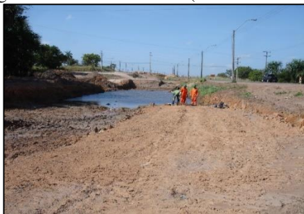
Figure 4. View of section 1 (Piles 181 to 188).
