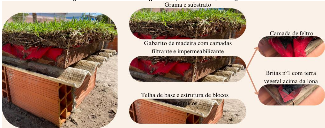
Image 2 - Schematic indicating each layer of the simplified green roof
