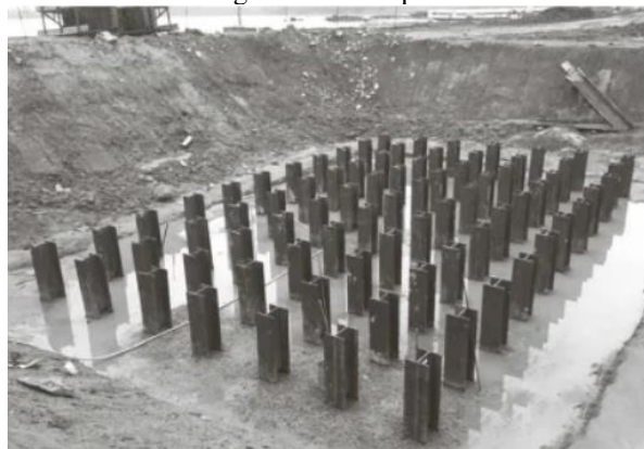
Figure 8 – Steel piles
