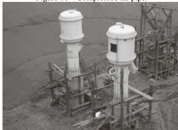
Figure 10 – Compressed air pipe.
