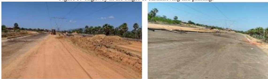
Figure 3. Highway in the stages of earthmoving and printing.
