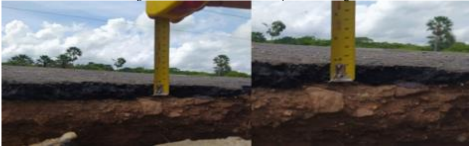
Figure 4. The thickness of asphalt coating
