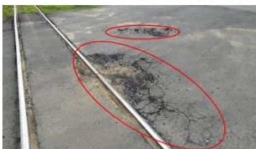
(c) Alligator leather cracks
