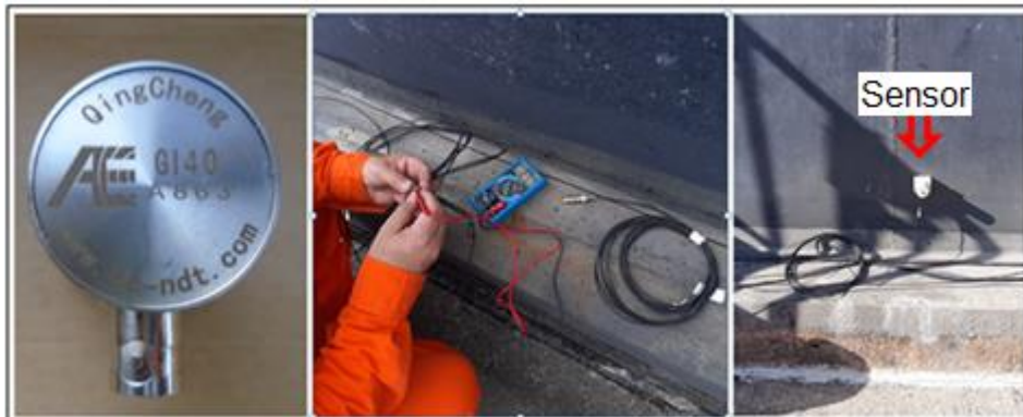
Figure 11 – Installation of piezoelectric sensors
