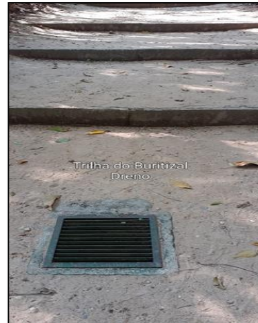
19 – Drain in the trail
