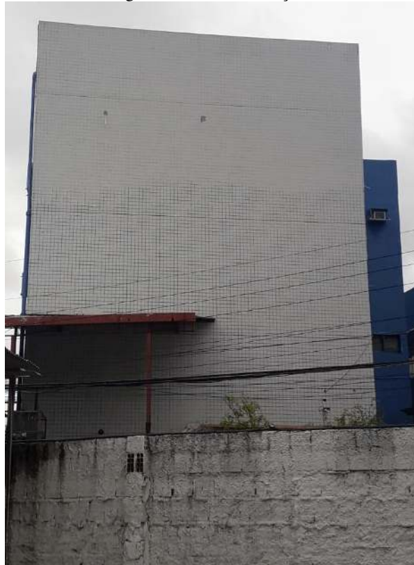
Figure 11 - Left side façade
