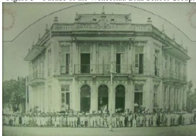
Figure 5 – Facade of the Wenceslau Braz School Group.
