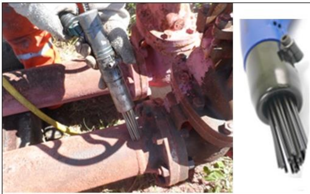
Figure 2. Action of the needle gun in the preparation of the metallic surface.
