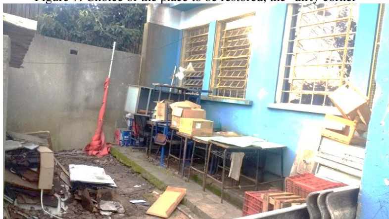
Figure 7: Choice of the place to be restored, the "dirty corner"
