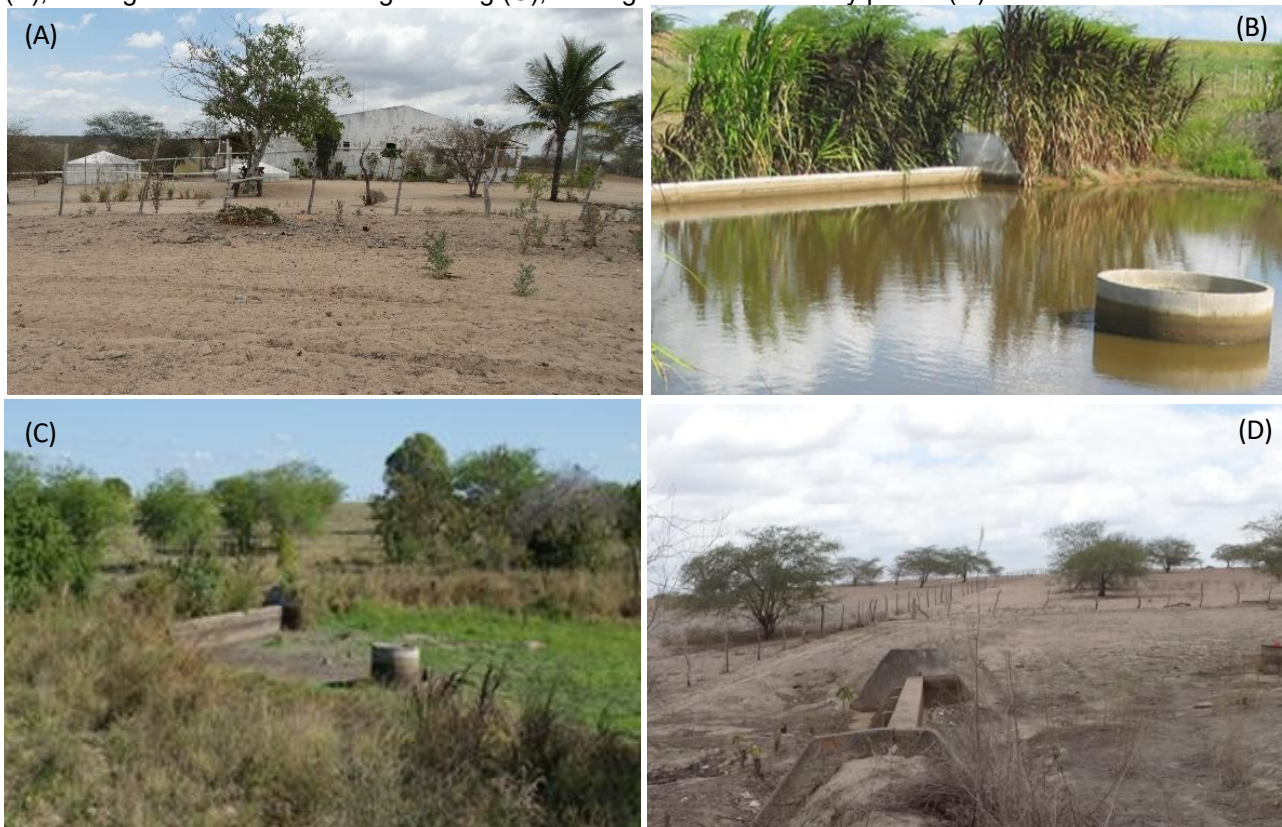
Figure 1. NSGA headquarters, Cacimbinhas Site (A); underground dam after first rains before water infiltrates (B); underground dam after forage cutting (C); underground dam in a dry period (D).
