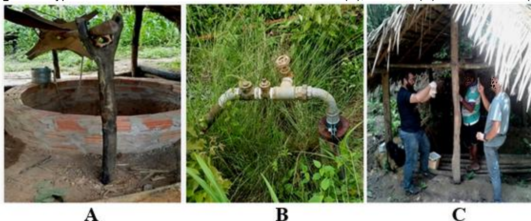
Figure 2. Types of Wells Used for Water Collection: Cacimba (A), Artesian (B) and Cacimbão (C).
