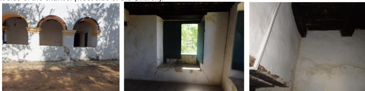
Figure 10: (left) – Attack by salts on the external west side façade. (center) – Attack by salts on the west side wall upper part (galleries above the balcony). (right) – Attack by salts on the inner wall of the Sacristy on the left side of the chancel (west side of the Church).
