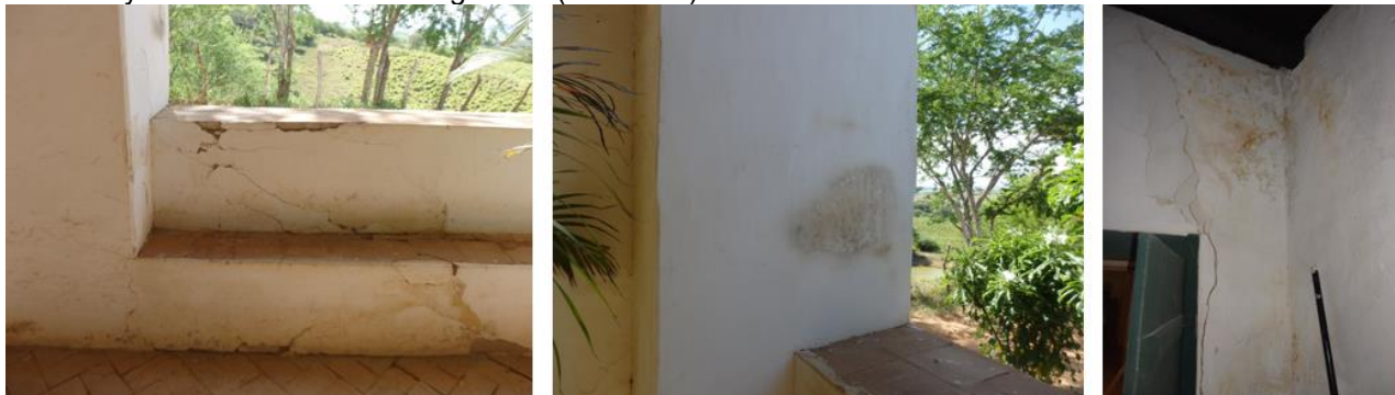
Figure 8: (left) – Humidity in the benches of the balcony of the west façade. (center) – Detail of infiltrations, moisture stain, balcony wall, west façade. (right) – Detail of condensation humidity accompanied by cracks in the sacristy on the left side of the high altar (west side).
