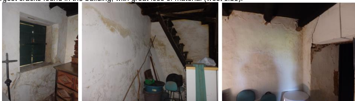
Figure 9: (left) – Internal side wall of the sacristy on the right side of the high altar (condensed humidity). (center) – Wall behind the high altar with high concentration of humidity and condensation. (right) – Detail of the internal wall of the sacristy on the left side of the altar, condensation humidity accompanied by one of the largest cracks found in the building, with great loss of material (west side).
