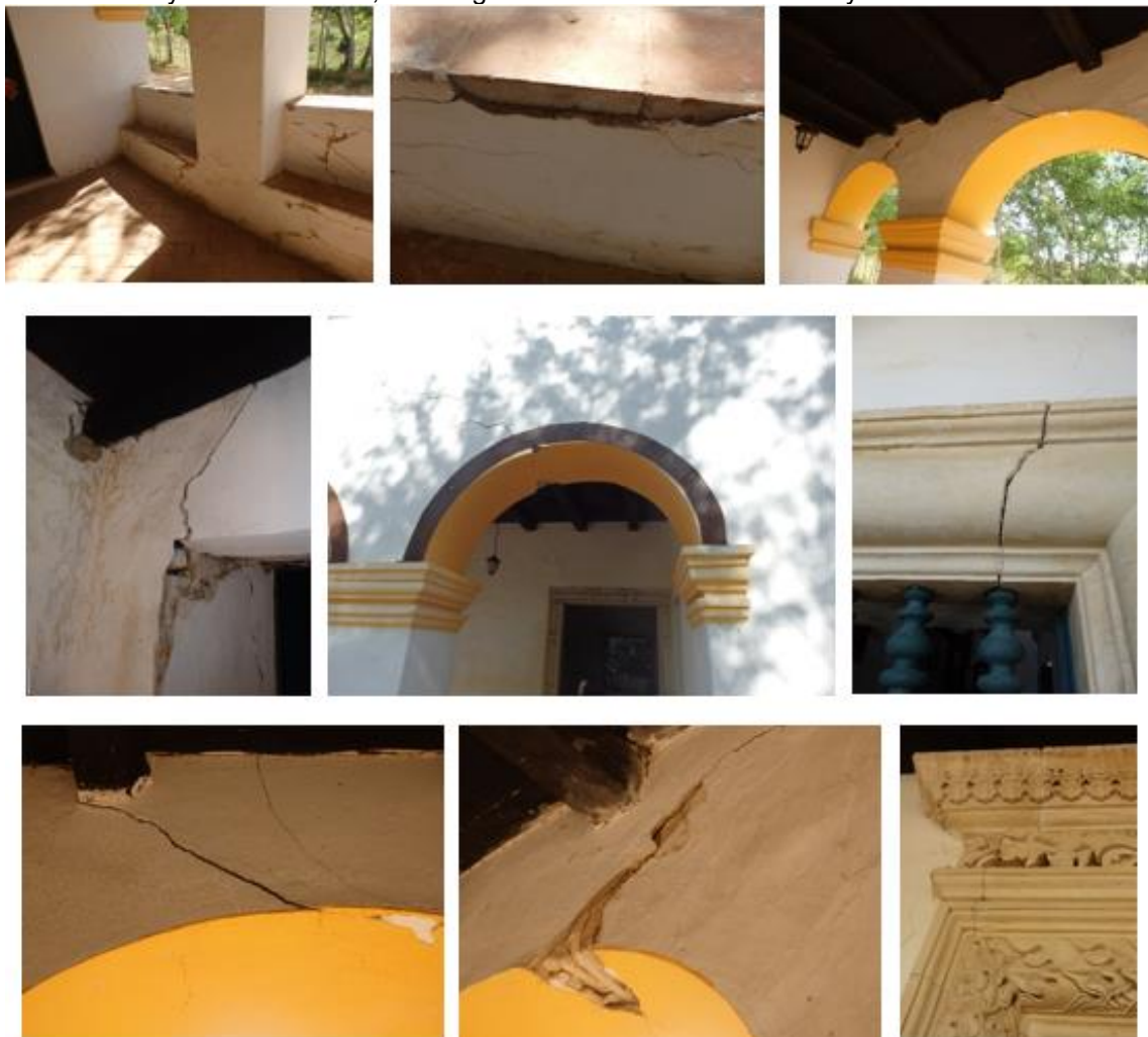
Figure 11: (above - from left to right) – Disaggregations, crushing and cracking in the benches and arches of the balcony of the west wall. (center - from left to right) – Crushing and cracking at the sacristy door; in one of the arches of the balcony with stabilization, both on the west wall; cracking in the limestone of the window next to the main doorway. (below - from left to right) – cracks with disaggregation and crushing in the center of the arches of the balcony of the west wall; cracking in the limestone main doorway.
