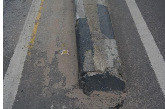
(c) Wheel guard with severe reinforcement corrosion (OAE 2)
